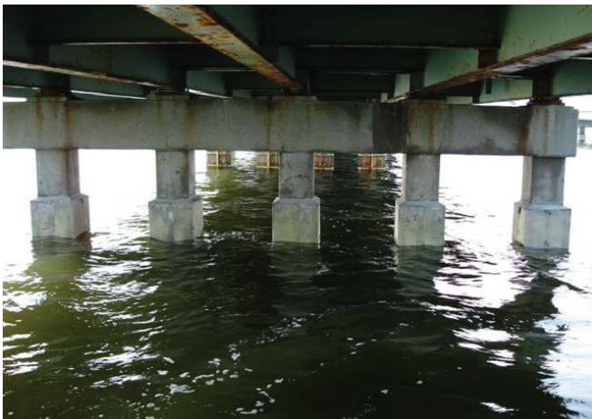
Galvanode DAS Marine Anodes inside stay-in-place FRP Forms
