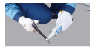
2. Cut the nozzle at the appropriate position diagonally.
