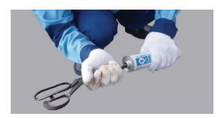
Break the moisture-proofing aluminium foil on top of the cartridge, and remove the metal back seamer from the bottom.
