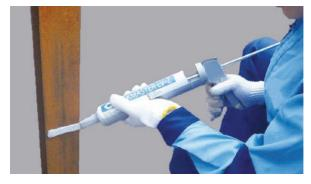
5. Apply Leakmaster continuously without a break to the place to be sealed.
