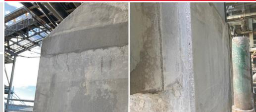
A break out and rebuild strategy was required to repair a structural concrete column supporting the sag mill concentrator. Being in the acid splash zone had led to concrete contamination and extensive re-bar damage. More than 20% of the steel reinforcement had to be replaced.
