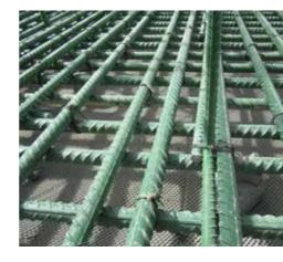
The structural steel reinforcement is laid directly on top of the membrane ready for the structural concrete placement.
