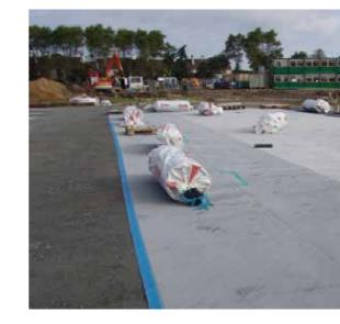
Blinding concrete is preferred, however Proofex Engage can be placed directly on top of a well compacted smooth granular fill substrate. A broadcast of damp sand on top of the granular material is useful.
