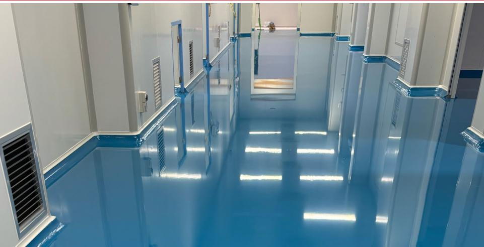
A durable, high gloss epoxy coating was required to upgrade the flooring in this busy pharmaceutical factory. Nitoflor FC150 HPSL offered application versatility plus high resistance to chemical attack and abrasion.
