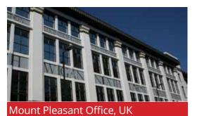
This landmark local building in London was suffering from the effects of old age cracking and carbonation. Fosroc's Renderoc repair system was able to repair the damage and re-profile the finish to a very high standard. The application of Dekguard E2000 provided durable and elastomeric protection, in the colour scheme desired by the designer.
