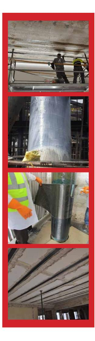
Fosroc Marine Jacket is a cathodic protection system provided specifically for marine piles. It is used on piers and jetties where the specific environment of high chlorides, moisture and oxygen combine adding erosion and mechanical abrasion into the mixture. This combination creates accelerated corrosion in the tidal and splash zones which is hard to combat using standard repairs and coatings.
